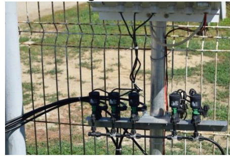
Fig. 7. Solenoid valves for irrigation plot selection
