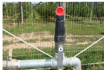
Fig. 3. Vent valve with tap
