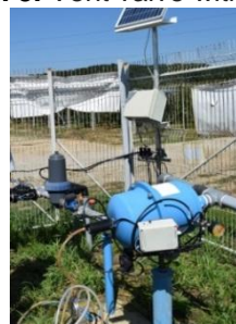
Fig. 3. Vent valve with tap
