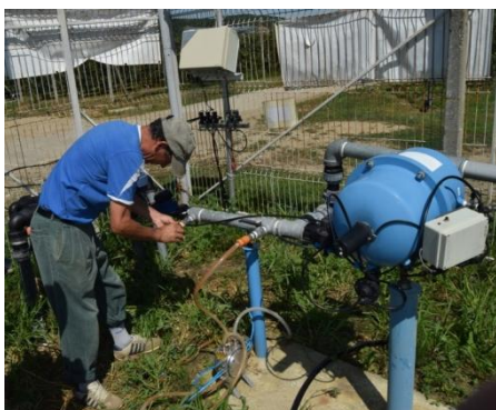
Fig. 8. Branching of the injection device to the local watering system
