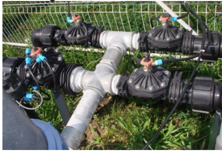
Fig. 7. Solenoid valves for irrigation plot selection
